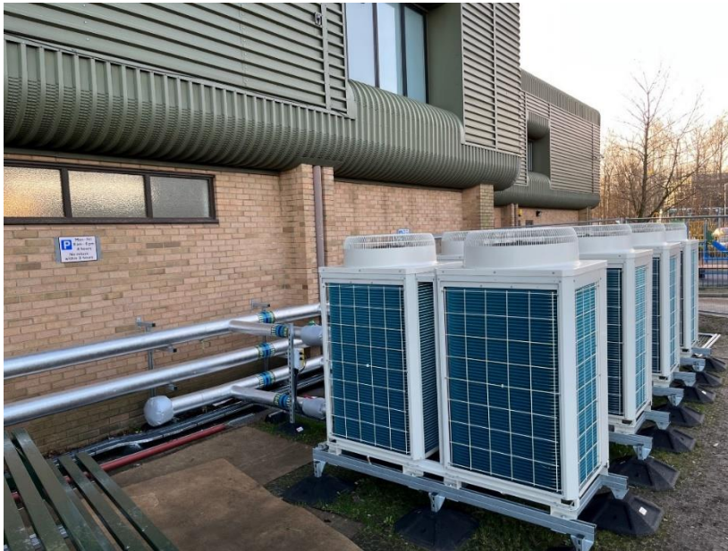
Image: Heat pumps providing heat to Abbey Leisure centre
