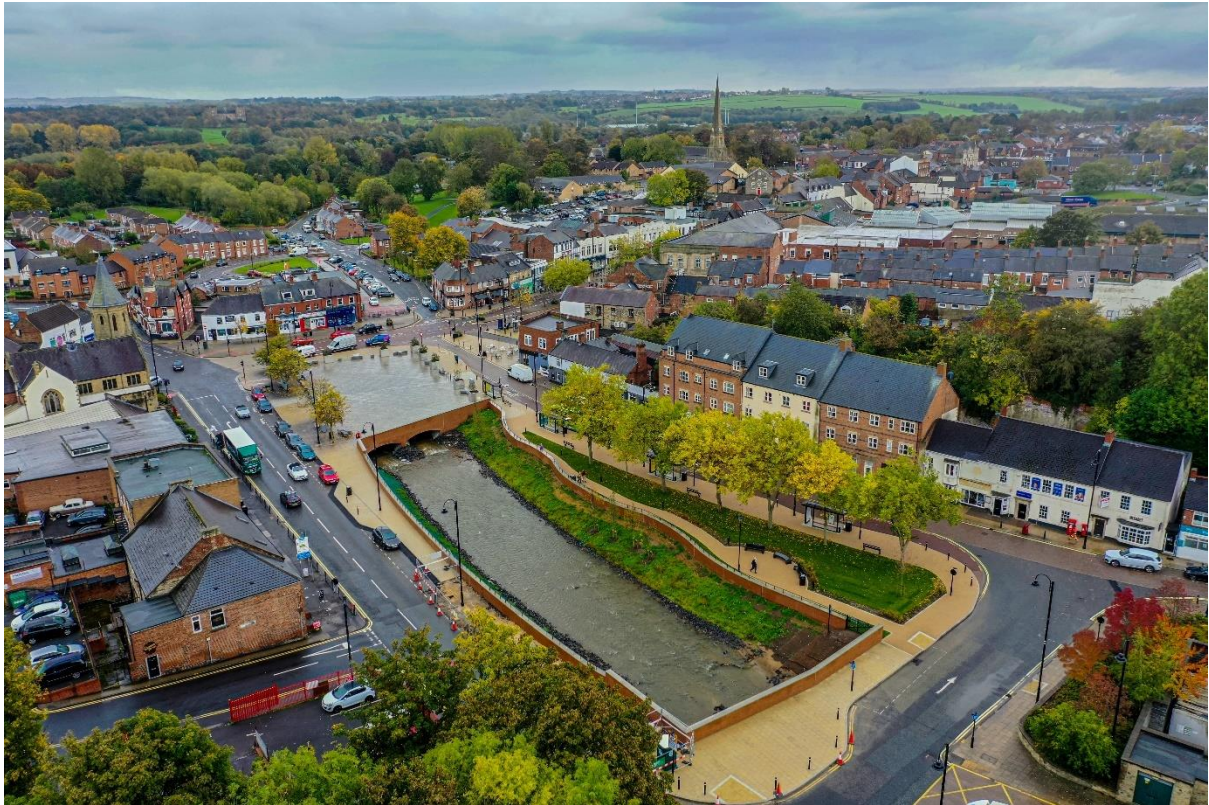
Chester-le-Street, Chester Burn de-culverting project.
